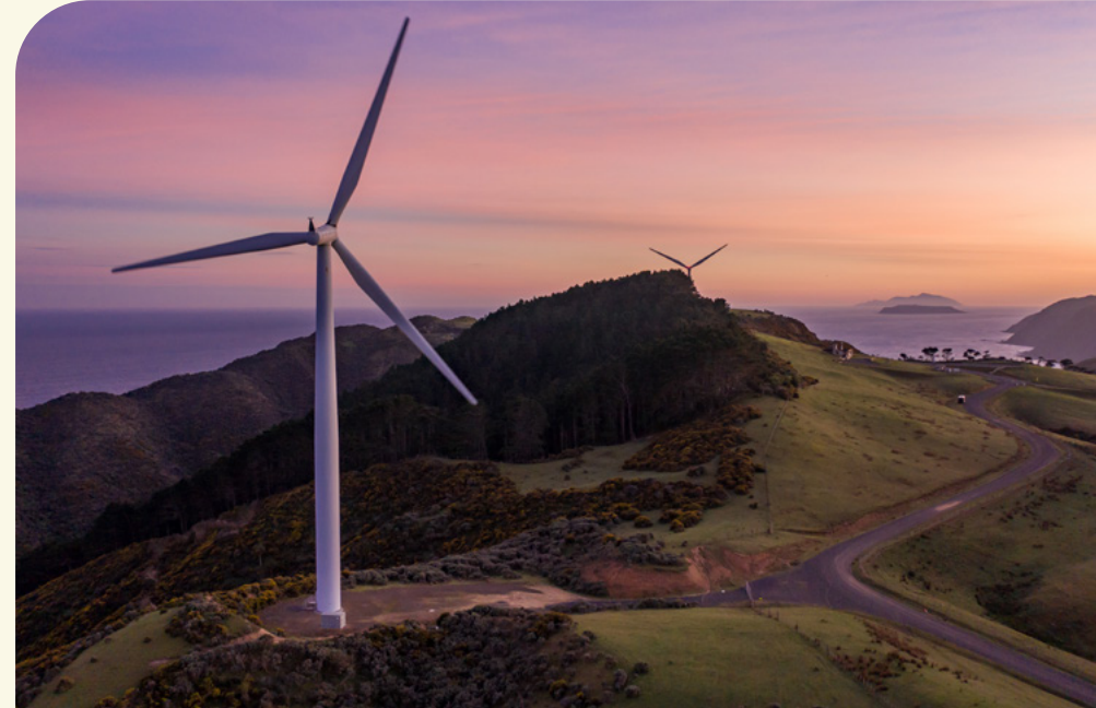
Meridian Energy's West Wind Farm, Wellington
